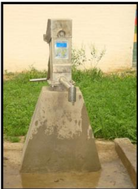
Figure 4: A Newly Installed Hand Pump by HOPE'87-Pakistan
