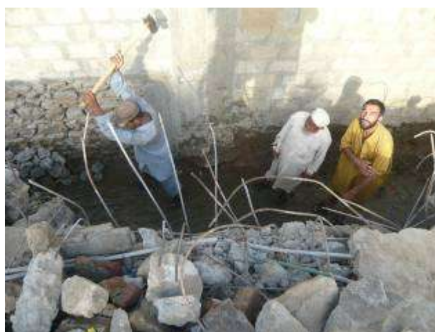
Picture7: Rehabilitation of Gullibagh Irrigation channel
